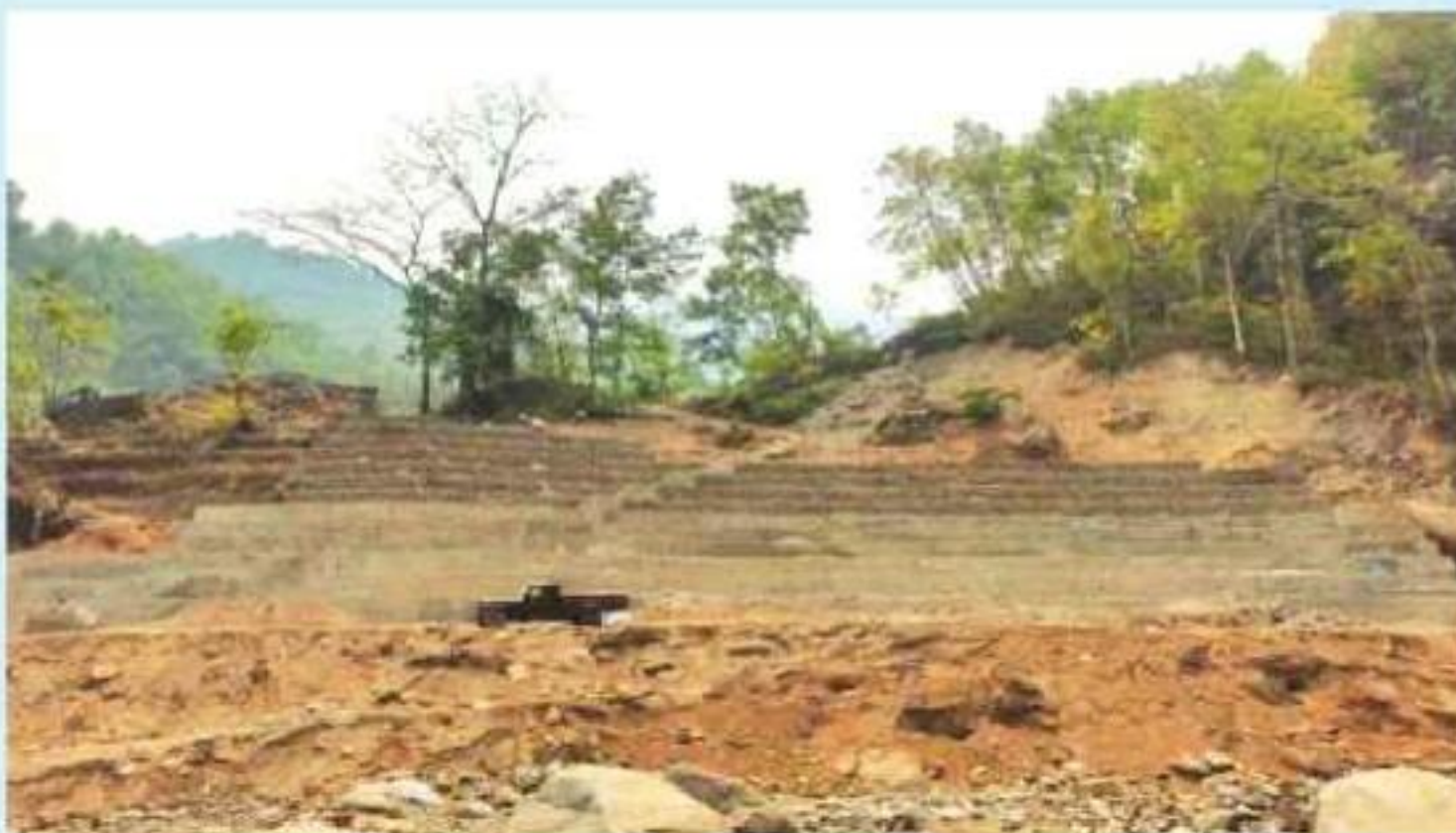
Protection wall at behind of switchyard
