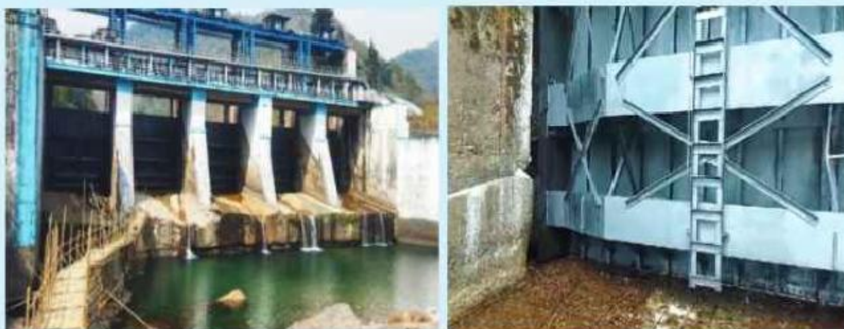
Barrage Gate at Bindu Barrage
