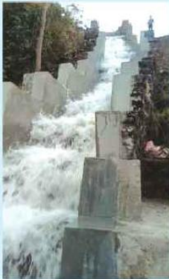
Chute drain from Forebay Silt Extruder (Chute drain in front of Adit-I of LICs) exit point to Anchor Block-5
