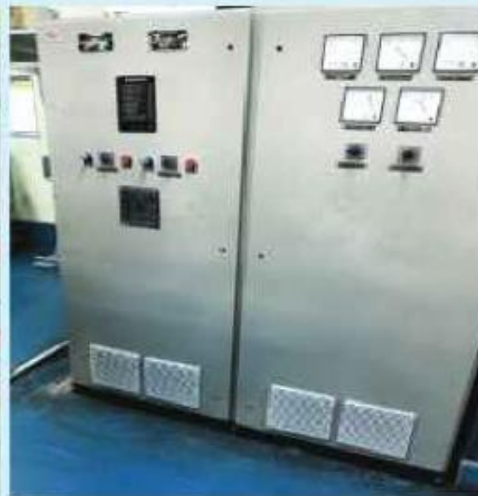
535 Ah Battery Bank and Battery charger
