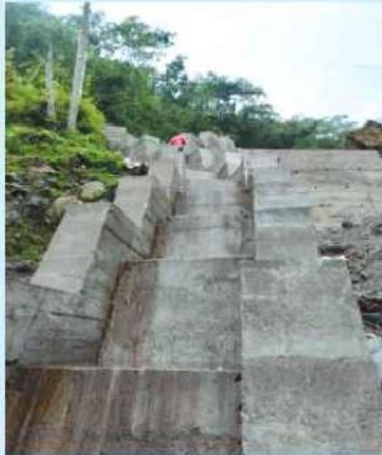
Chute drain from Forebay Silt Extruder (Chute drain in front of Adit-I of LICs) exit point to Anchor Block-5
