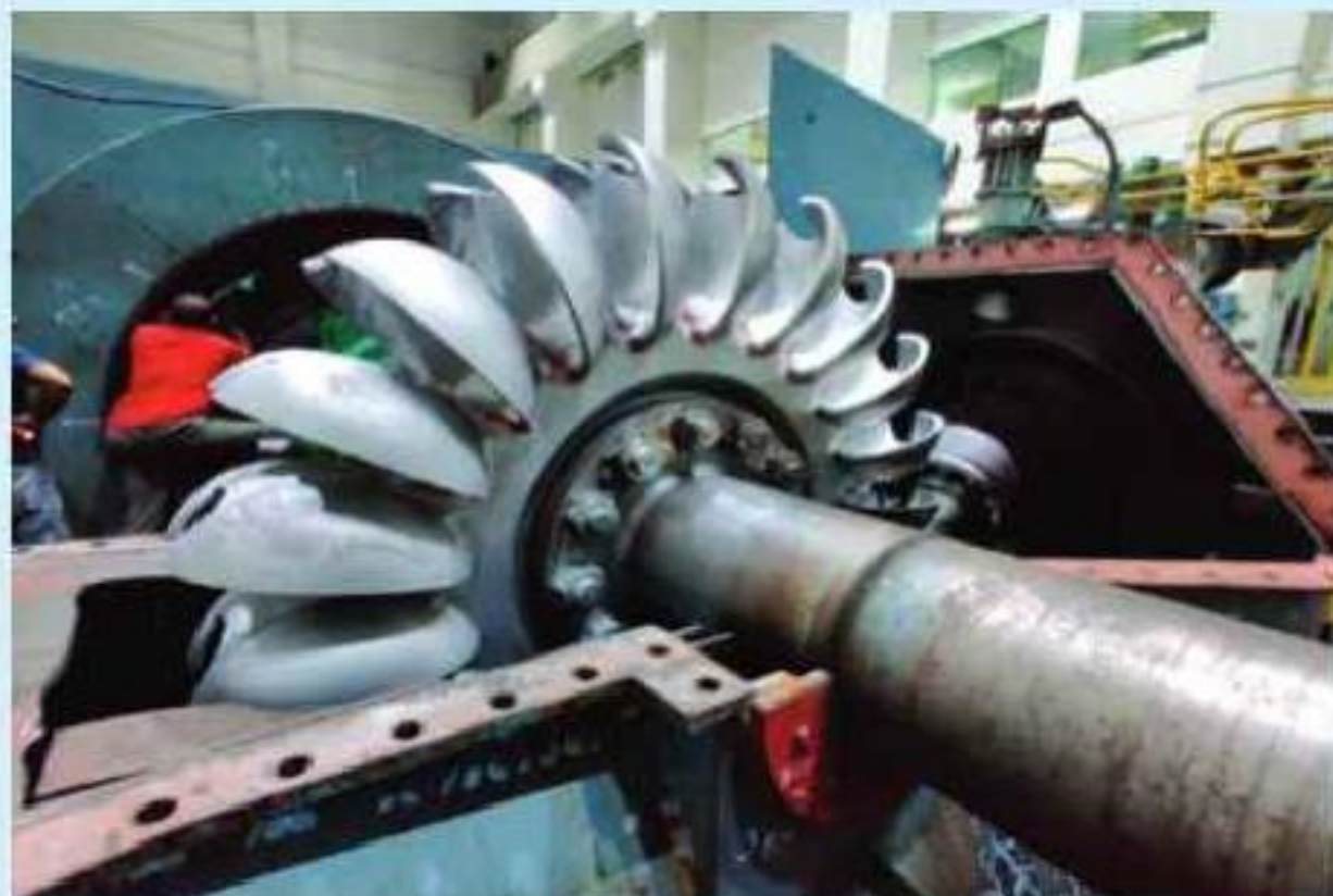
Unit No.4 runner replacement
