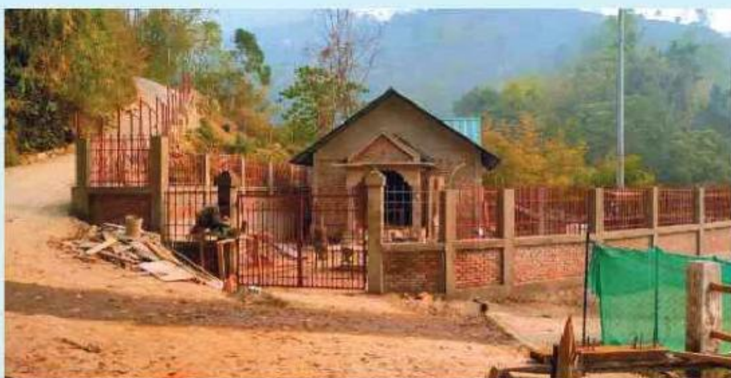
Construction of Sidrapong Museum
