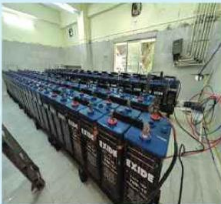
535 Ah Battery Bank and Battery charger
